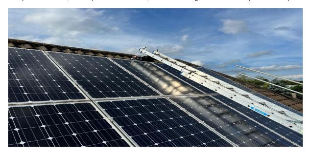
The edges of all the panels were cleaned using biocide, to not only sterilise the area, but by having clean edges on each panel, this ensures a good surface for the adhesive that will be applied to each strip of plastic proofing. A clean surface makes for a very strong bond once this is applied.
